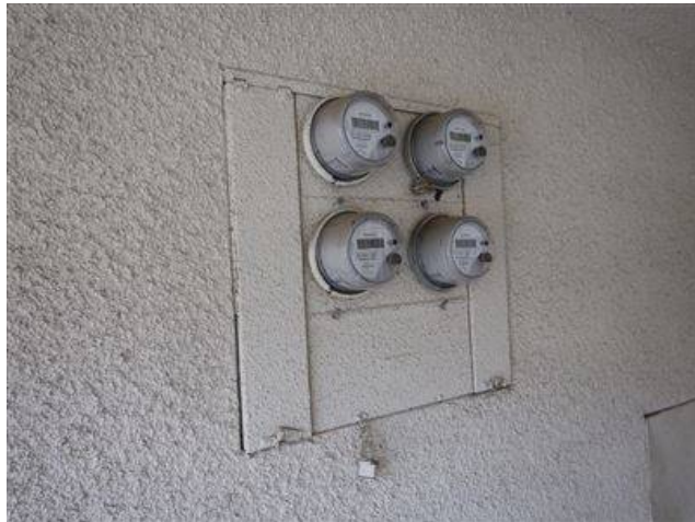
Photo 5-2 NEXT TO THE CRAWL SPACE ACCESS POINT
