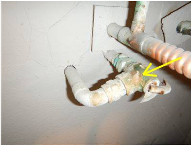
Photo 6-1 LOCATED ABOVE THE WATER HEATER
