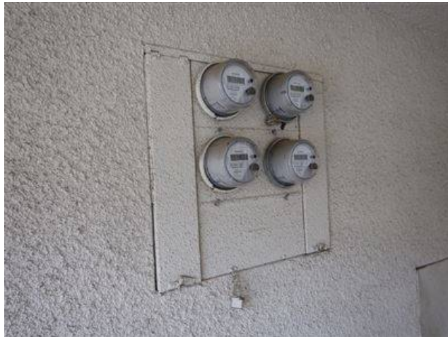
Photo 5-2 NEXT TO THE CRAWL SPACE ACCESS POINT
