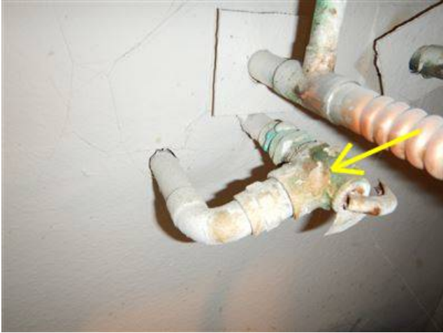
Photo 6-1 LOCATED ABOVE THE WATER HEATER
